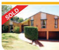
Wisteria Crescent, Cherrybrook
